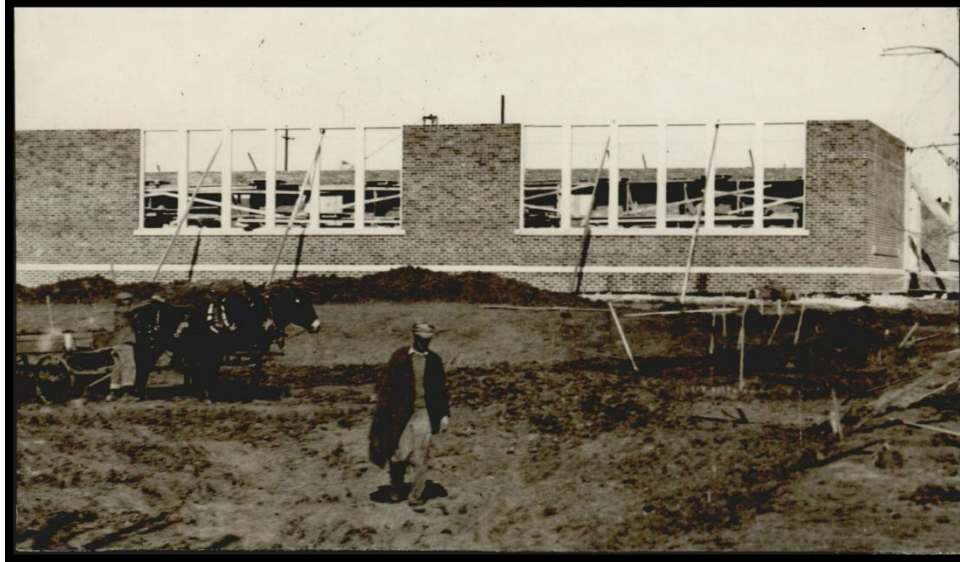
Construction Photograph of Creston Hills Elementary School used for a story in the Oklahoma Times newspaper. Caption: "Construction financed by P W A" Oklahoma Times, Oklahoma City, Oklahoma, January 26, 1934
