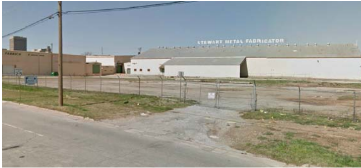
The Steel Yard / East Bricktown Hotel Site Location Before
