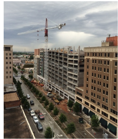
Garage Nearing Completion (7/2014)
