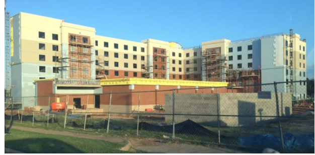
OU E-Suites Hotel Mid-Construction (07/2014)
