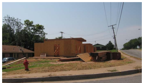
SE Corner of 10 th & Lottie (Framing Underway)
