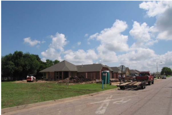
1709 NE 6 th (Fairhaven) Under Construction
