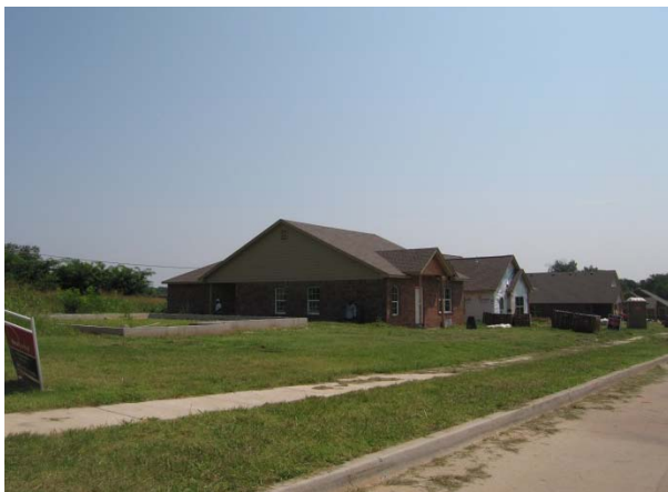
1701/05/09/13 Euclid, (Affordable Units Under Construction)
