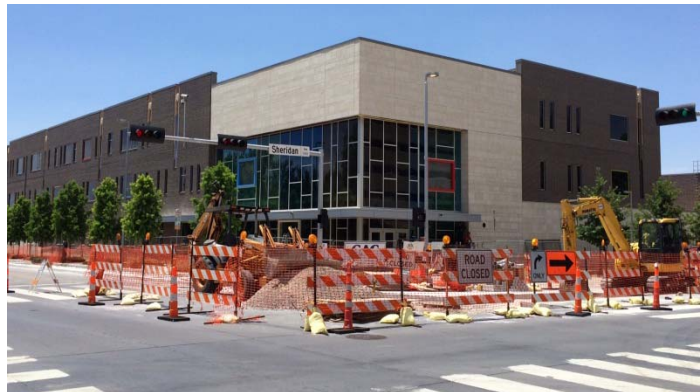
John Rex Elementary School Mid-Construction (7/2014)
