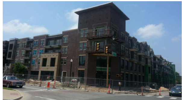
The Edge Mid-Construction (7/2014)
