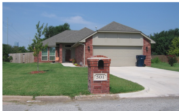
501 N. Bath Ave. Market Rate Home Completed
