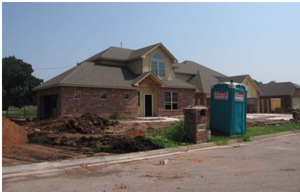
1701/03/05 NE 6 th (Fairhaven Triplex) Under Construction
