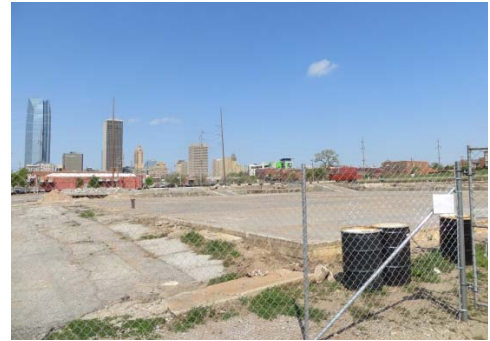
The Steel Yard / East Bricktown Site Cleared
