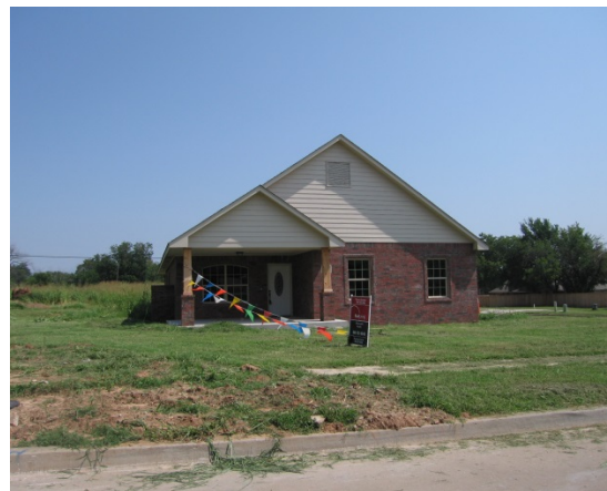
1701 Euclid (Nearing Completion)
