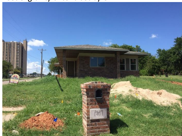
Construction Underway on Home
