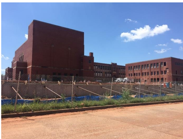
Site Under Construction
