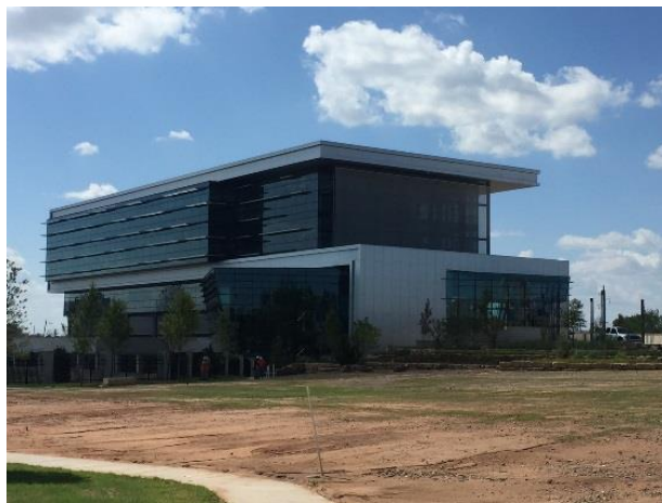
GE Research Center Nearing Completion
