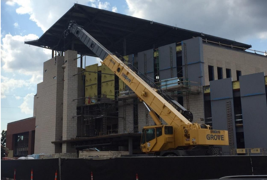
Municipal Court Building Under Construction
