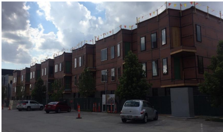
Civic Centre Flats Under Construction
