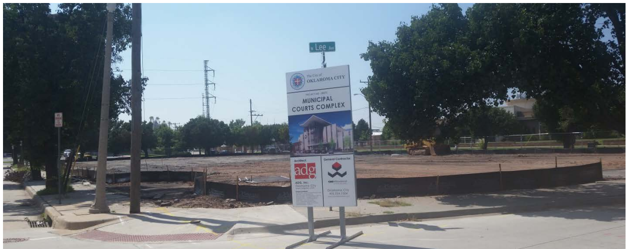
New Municipal Court Site Before
