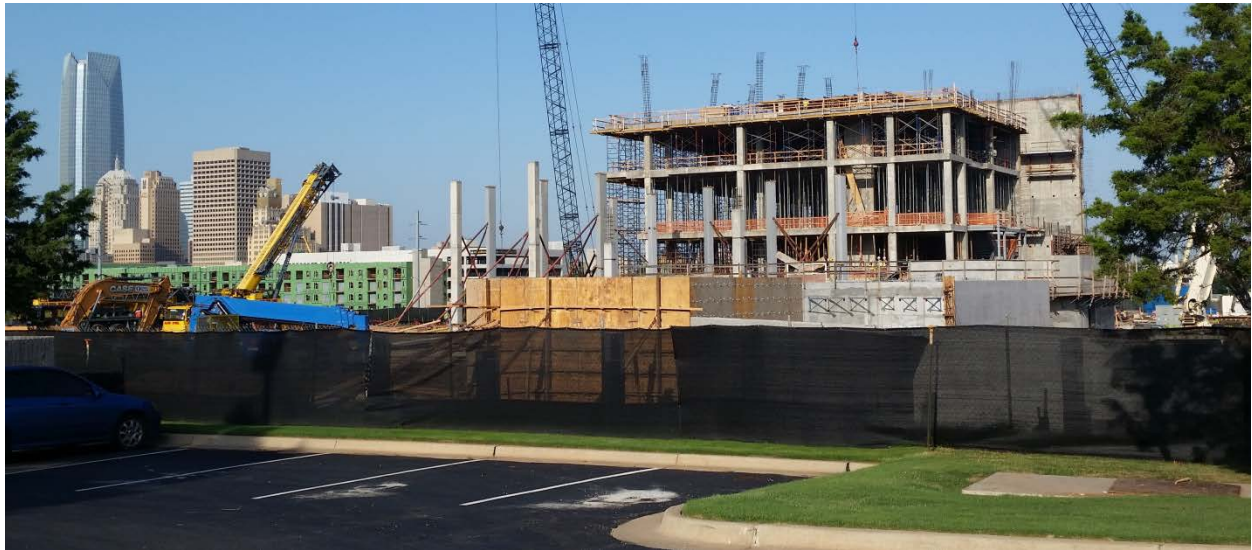
GE Research Center Site Under Construction
