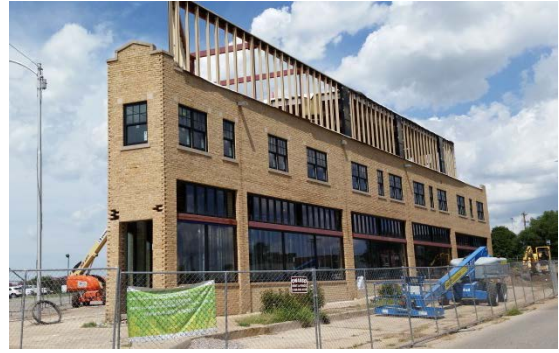
Flatiron Triangle Building Mid-construction
