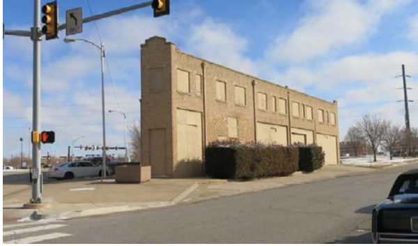
Flatiron Triangle Building Before
